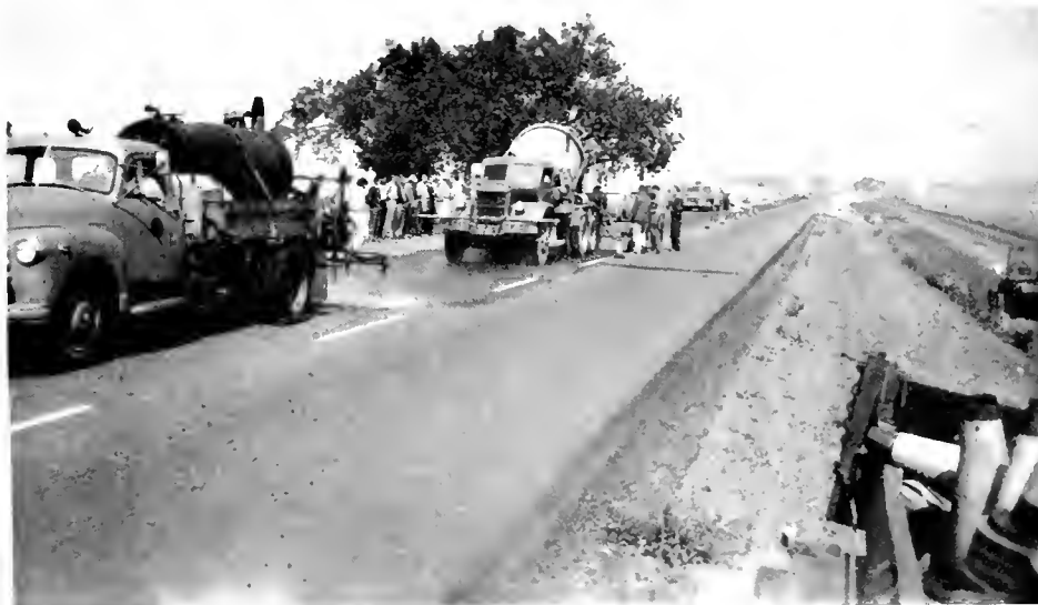
Slurry train in action
